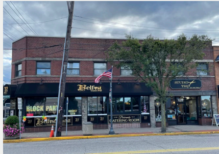
Existing Façade Conditions
