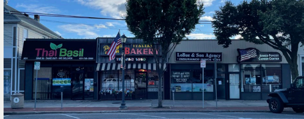
Existing Façade Conditions
