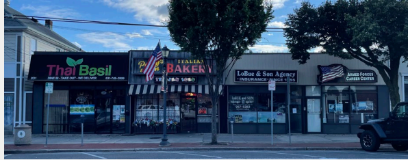
Existing Façade Conditions
