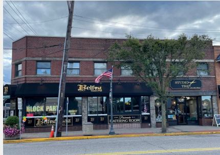
Existing Façade Conditions
