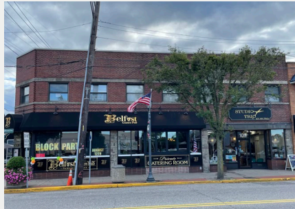
Existing Façade Conditions
