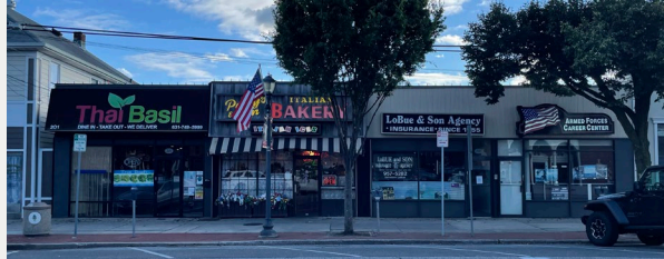
Existing Façade Conditions
